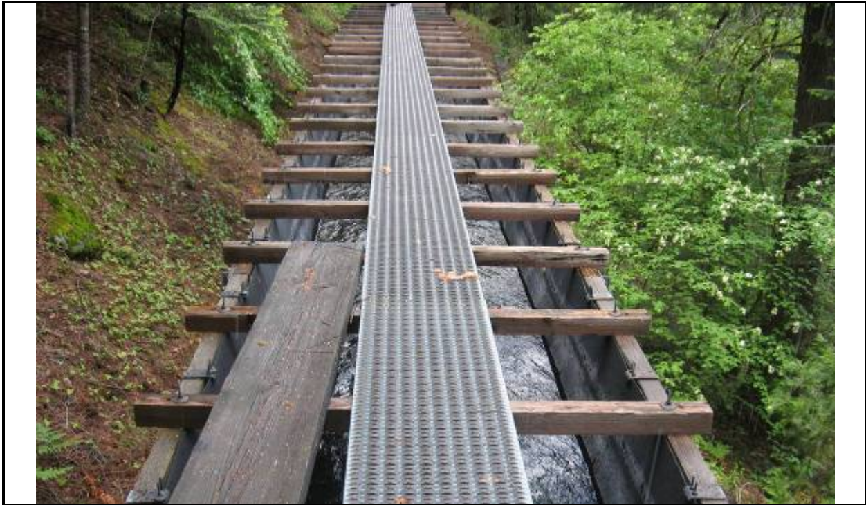
Photograph A-7. Wooden Flume Section of Kilarc Main Canal.
