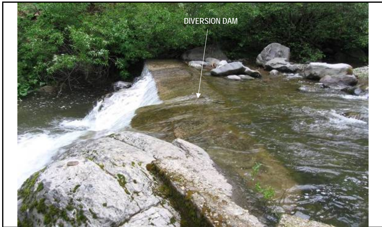
Photograph A-3. Kilarc Main Canal Diversion.
