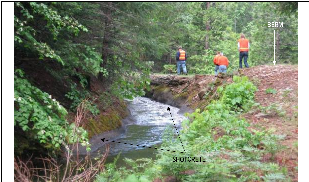
Photograph A-6. Shotcrete Lines Section of Kilarc Main Canal.
